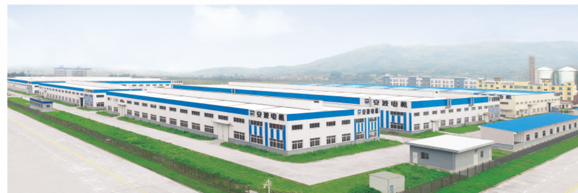
▪ 宁德工厂 Ningde Factory
