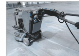
地坪研磨 Floor grinding equipment
